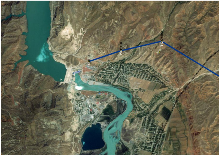
Figure 2-3: Sangtuda Hydropower Station
